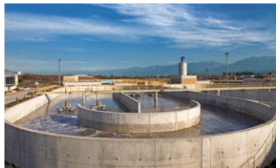
Every day, REMONDIS processes up to 80,000 cubic metres of water at each of the facilities under its control
